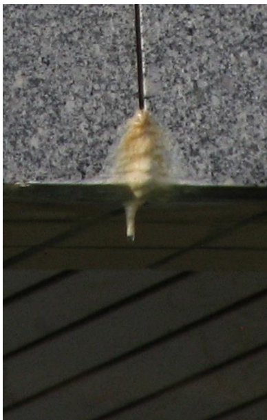
Figure 3. Example of calcium carbonate neoformation with stalactite-like structure on a granite slab (if you look closely you might be able to see on the lower tip of the "stalactite" a drop of the solutions that are forming it).
