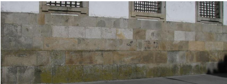
Figure 8. A wall with regular distribution of regular shaped stones (it is possible to define referencing for locating individual stones and individual features inside a given stone).
