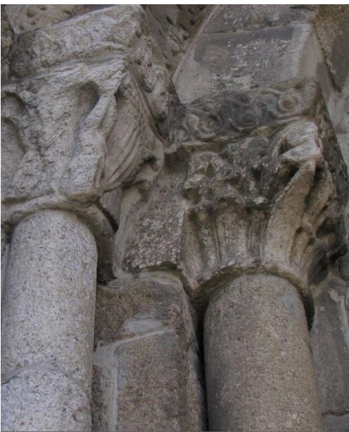
Figure 5. Image of two granite types on columns of a portal in a monument of Braga (NW Portugal): the darkish-brownish one on the right is similar to the local granite while the lighter one on the left is similar to certain facies from surrounding regions.
