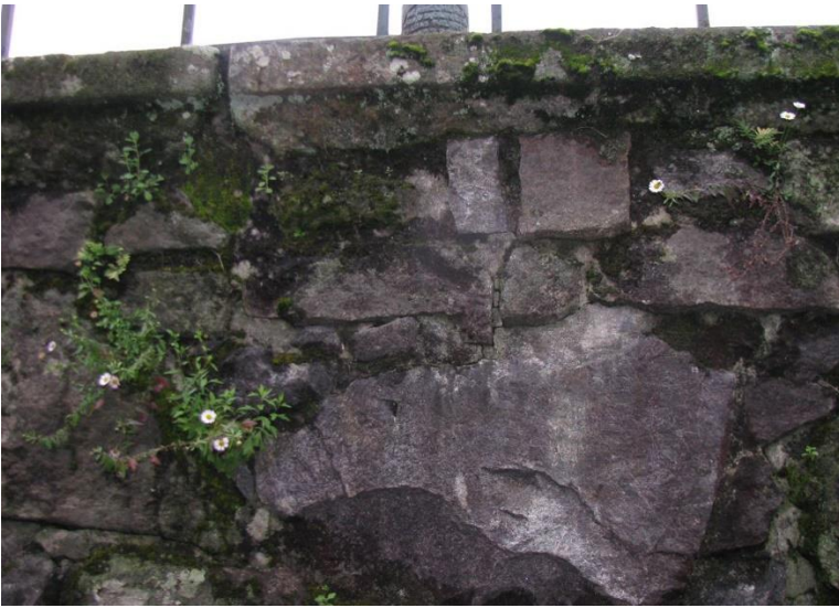
Figure 4. Illustrative image of relations between substrate and biological colonization with lichens and moss on the stones and plants in the joints between the wall stones.
